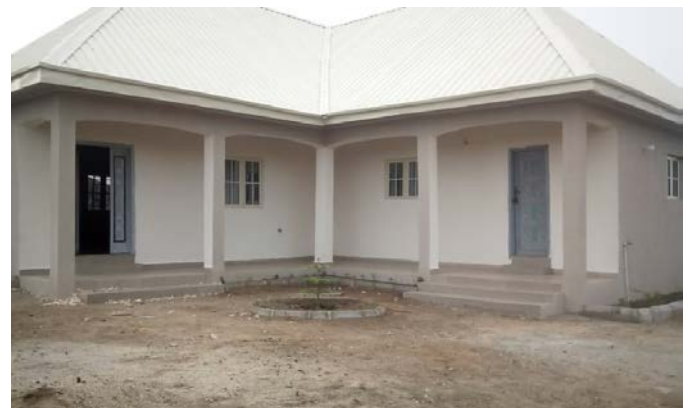
Picture of the nearly completed Skills Center, ready for occupancy after the Covid-19 shutdown is lifted.
